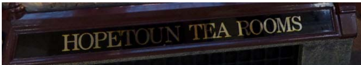
Glass Panel Located on (LEFT) Side of Tenancy – installed after 1975
